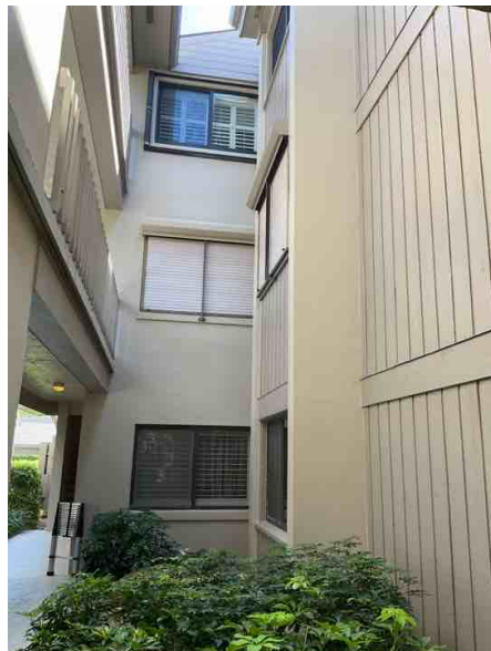
Elevation and unprotected glazed openings
