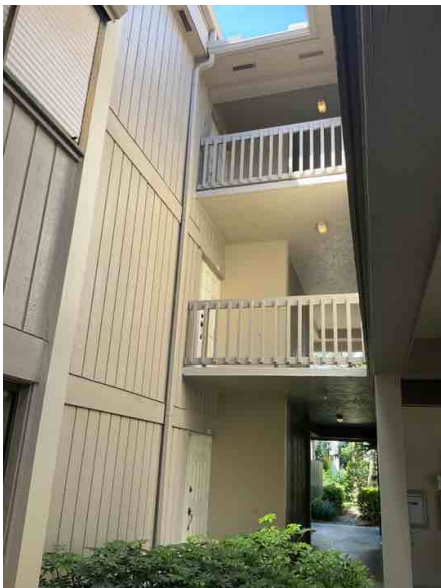
Elevation and unprotected glazed openings
