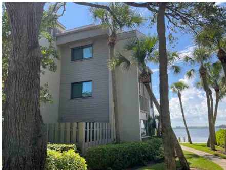
Elevation and unprotected glazed openings
